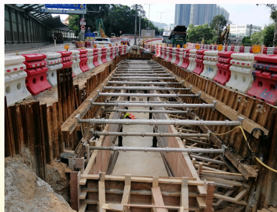
蔚景園對出中央分隔帶位置興建樁帽 Pile cap construction works near Scenery Court at central median
