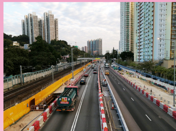
豐和邨對出中央分隔欄安裝護欄以便行車線改道 Installation of highway guard for road lane shifting at central divider near Fung Wo Estate
