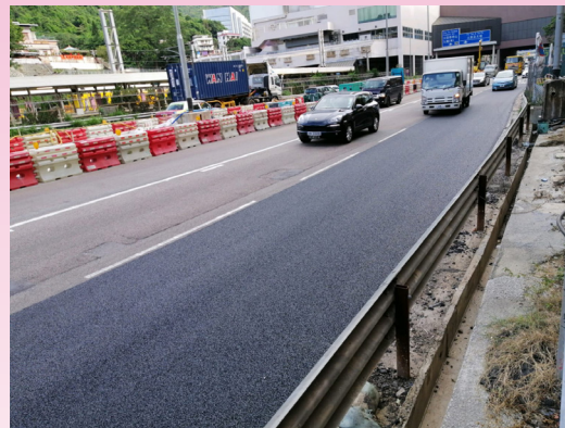
拆除偉華中心對出鐵板和復原臨時路 Removal of steel plate and reinstatement of temporary road in front of Wai Wah Centre
