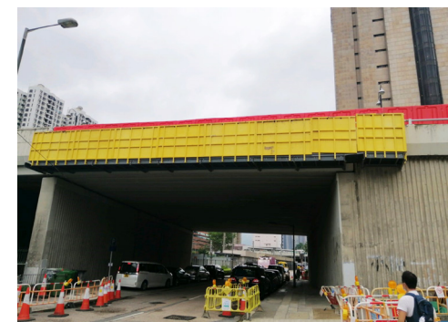
沙田鄉事會路興建工作台 Construction of temporary working platform on Sha Tin Rural Committee Road
