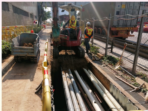
遷移近偉華中心對出單車徑的地下設施 Utility diversion on cycle track near Wai Wah Centre
