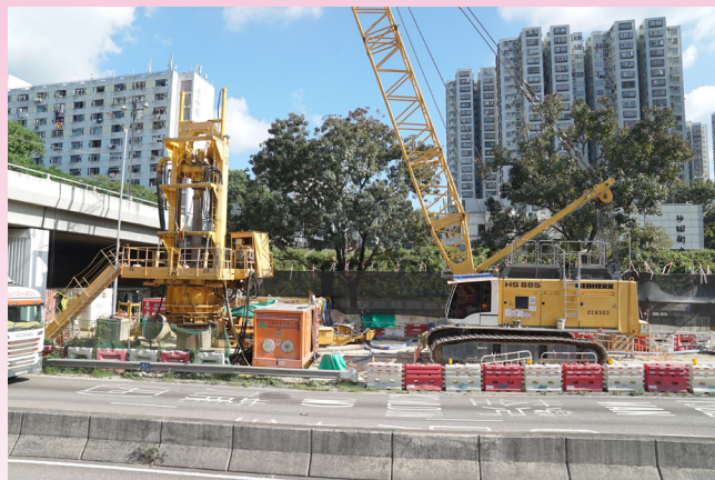
沙田鄉事會路支路旁興建鑽孔樁 Construction of bored pile alongside slip road of Sha Tin Rural Committee Road
