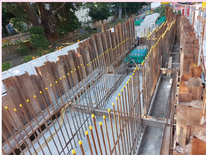
大埔公路近禾輦邨進行隔音屏障地基工程 Construction of noise barrier foundation along Tai Po Road near Wo Che Estate
