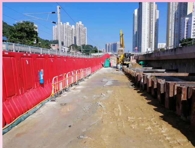
沙田鄉事會路支路興建護土牆 Construction of retaining wall alongside slip road of Sha Tin Rural Committee Road
