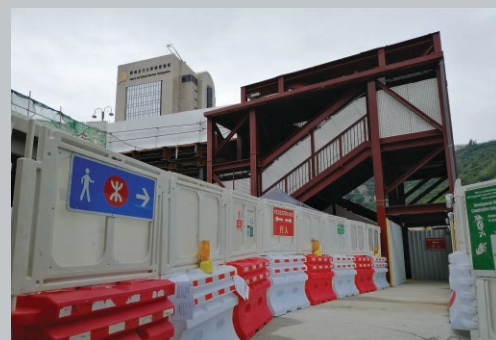
興建臨時通道樓梯準備改建沙田鄉事會路行人通道 Construction of temporary access staircase for diverting walkway of Sha Tin Rural Committee Road
