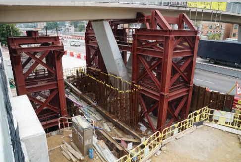
改建禾輦街行人天橋橋墩 Modification of the piers of footbridge on Wo Che Street
