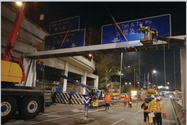
拆除鄰近連城廣場的架空標誌架 Removal of Sign Gantries near Citylink Plaza
