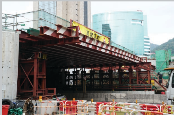
建造設有4.6米高度限制工作台 以用作沙田鄉事會路改建工程 Erection of working platform for Sha Tin Rural Committee Road modification works with the implementation of 4.6m height restriction
