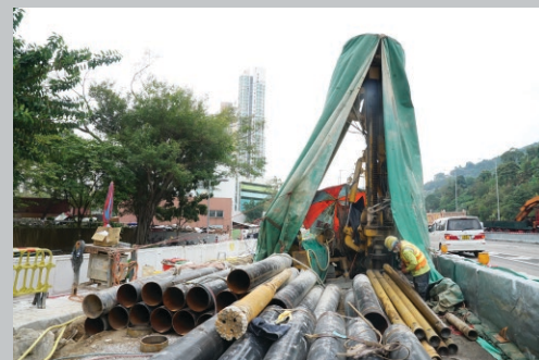
鄰近火炭路路肩位置興建迷你樁 Mini-pile construction near Road Verge of Fo Tan Road
